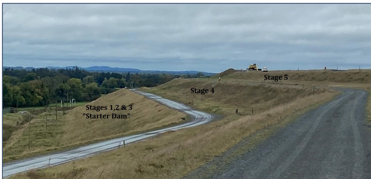
Figure 3.6 Existing Embankment Walls
